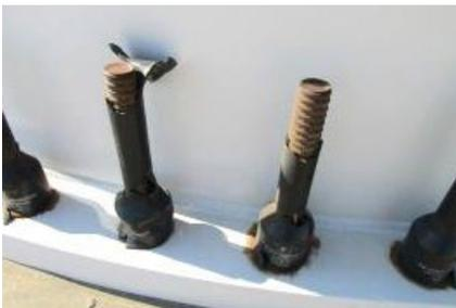
**Anchor Bolt Maintenance:** Anchor bolt tensioning procedures should be in place to periodically confirm that the anchor bolts are tensioned in accordance with the foundation design technical specifications. Procedures should indicate an interval for inspection and provide a means for technicians to classify and remediate any anchor bolt corrosion.
