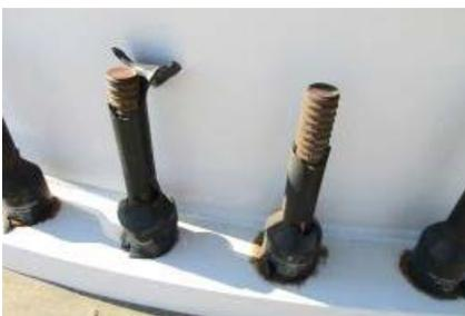
**Anchor Bolt Maintenance:** Anchor bolt tensioning procedures should be in place to periodically confirm that the anchor bolts are tensioned in accordance with the foundation design technical specifications. Procedures should indicate an interval for inspection and also provide a means for technicians to classify and remediate any anchor bolt corrosion.
